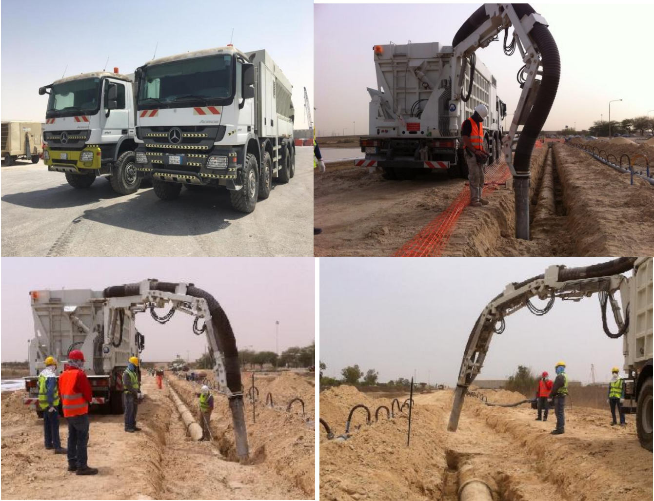
2 Units - Vacuum Excavators (Year 2013)
